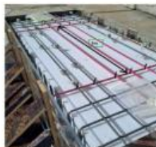
UHPC (floating Fiber Optic bars and sensors)
